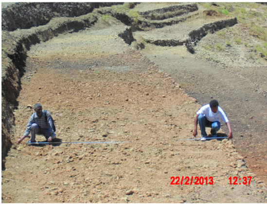
Bench Terraces under construction (left) and under cultivation (right) (Images Courtesy: Mekelle University)
