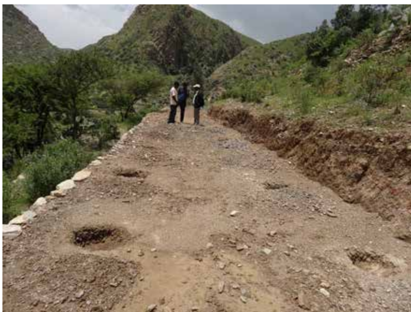
Plate 13. A bench terrace constructed as a demonstration in Gule watershed, Ethiopia (funded by Wukro Saint Mary College) (picture: Kifle Woldearegay).
