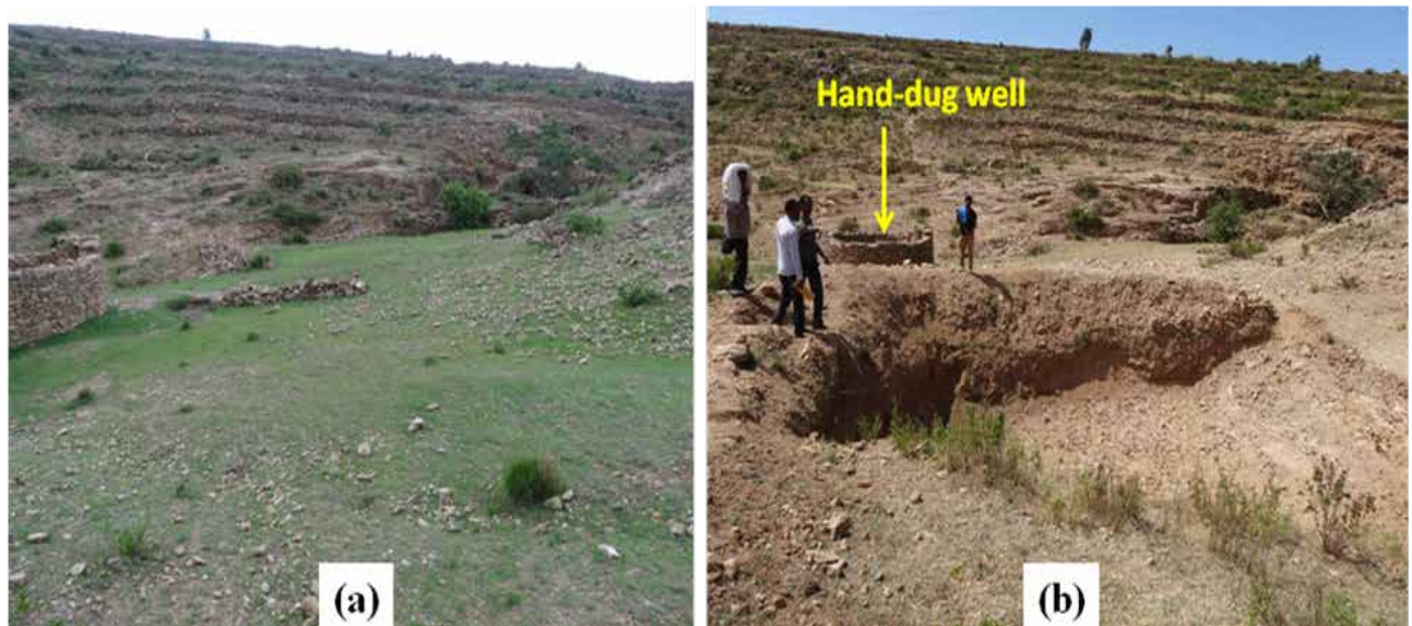
Plate 5. A percolation pond (12m long, 8m wide and 2m deep) constructed in the month of August 2013 has contributed to the enhancement of shallow groundwater (hand-dug wells) at downstream areas as well as reduction in erosion and surface runoff, Gule watershed, Ethiopia: (a) before construction, and (b) after construction of the percolation ponds (pictures: Kifle Woldearegay).
