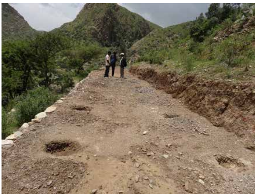
Plate 13. A bench terrace constructed as a demonstration in Gule watershed, Ethiopia (funded by Wukro Saint Mary College) (picture: Kifle Woldearegay).
