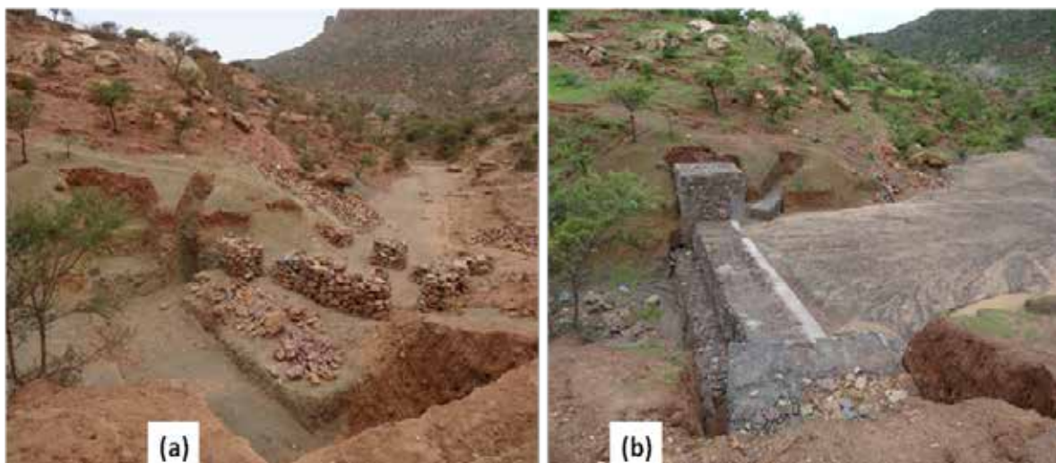
Plate 7. Gabion check-dams which are constructed to rehabilitate degraded streams and to enhance groundwater recharge in Gule watershed, Northern Ethiopia (project is funded by WFP through TBoARD) (pictures: Kifle Woldearegay).
