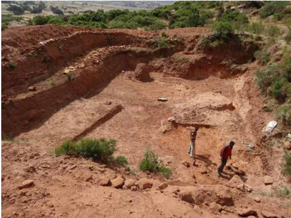
Plate 6. Percolation pond (20m long, 15m wide and 2.5m deep) constructed to recharge the shallow groundwater system and enhance spring discharge at downstream areas which could be used for small-scale irrigation (picture: Kifle Woldearegay).
