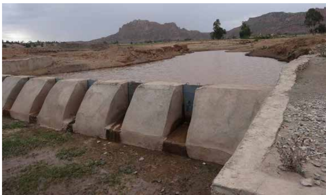
Plate 8. Check-dam pond which is constructed to store/diver stream flow for irrigation and shallow groundwater recharge in Gule Watershed, Northern Ethiopia (project is funded by REST) (picture: Kifle Woldearegay).
