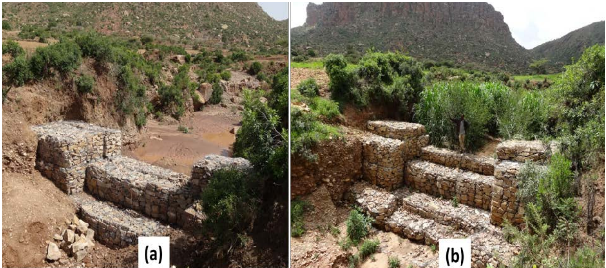
Plate 4. Gabion check-dams which are constructed to rehabilitate degraded streams and to enhance groundwater recharge in Gule watershed, Northern Ethiopia (project is funded by Wukro Saint Mary College): (a) before biological treatment in July 2013 and (b) after biological treatment in July 2014.
