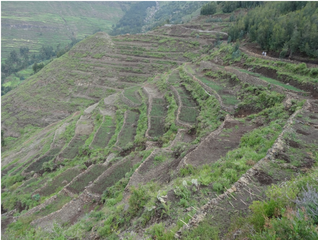
Plate 9. Bench terrace developed and distributed to local youth in Embahazti, Tigray, Ethiopia (note: bench terrace is constructed in 2013) (Photo: Kifle Woldearegay).
