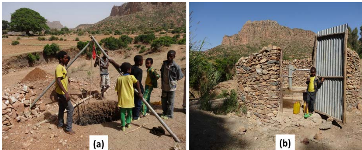
Plate 6. Shallow hand-dug well downstream of the gabion check-damps and percolation ponds: (a) during the excavation of the well, (b) the same hand-dug well which became productive throughout the year after, Ethiopia.
