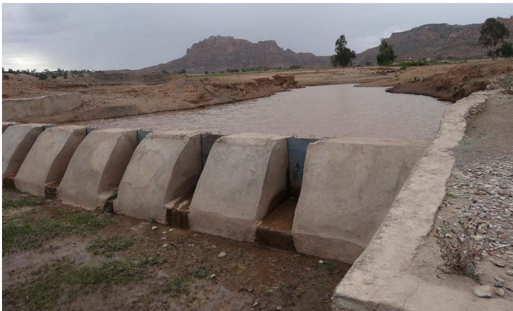
Plate 5. Check-dam pond which is constructed to store/diver stream flow for irrigation and shallow groundwater recharge in Gule Watershed, Northern Ethiopia (project is funded by Relief Society of Tigray).
