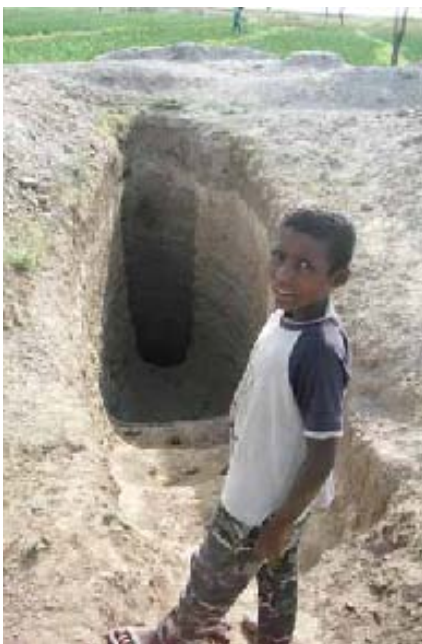
Figure 2. Dugwells in flood plains: prone to collapse and vulnerable to lowered water tables (Photo credit: MetaMeta)
