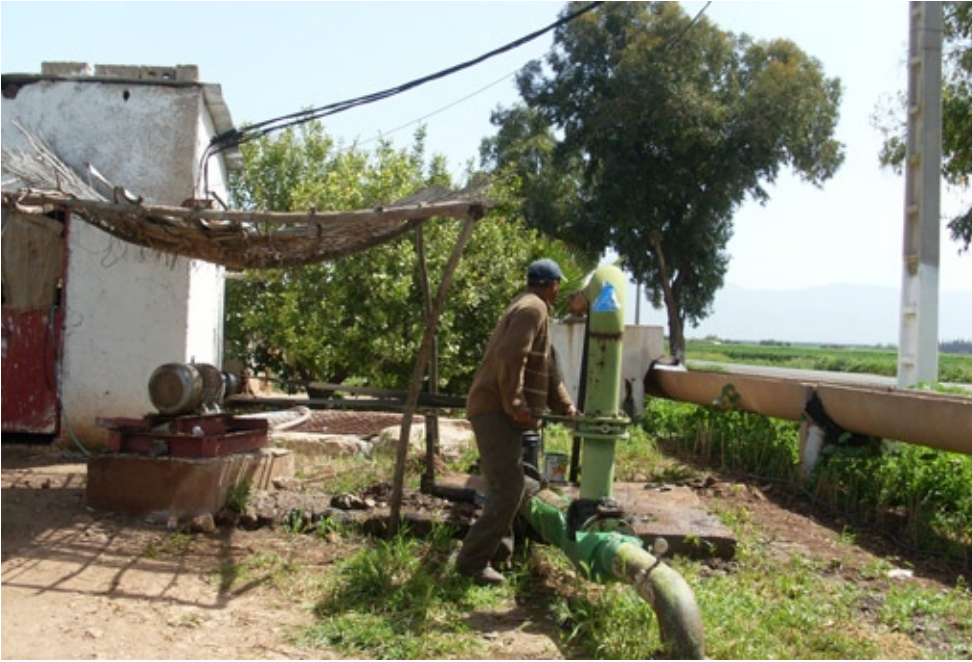
Figure 1. Using groundwater and surface water for irrigation purposes in Morocco
