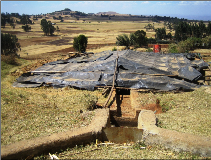
Figure 2. Rainwater harvesting structure with intake structure, silt trap and plastic roof
