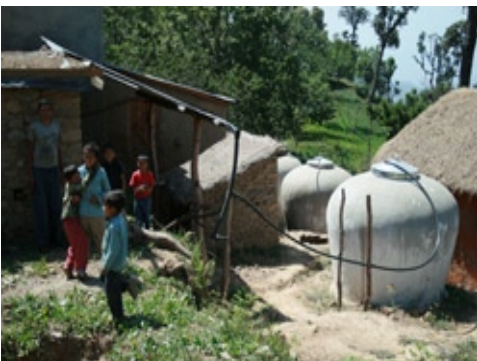
Figure 1. Rainwater harvesting tanks in Bubeyrakhe, Nepal
