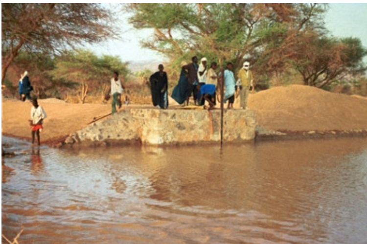
Figure 4. flood flow entering the infiltration basin
