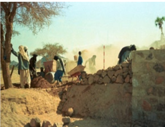
Figure 2. Construction of diversion works
