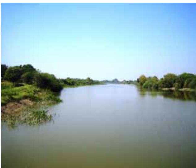
Figure 2 and 3. Piers with installed shutters and bridge (upper) Reservoir area upstream of KTW (below) (Photo credit: Olaf Verheijen)
