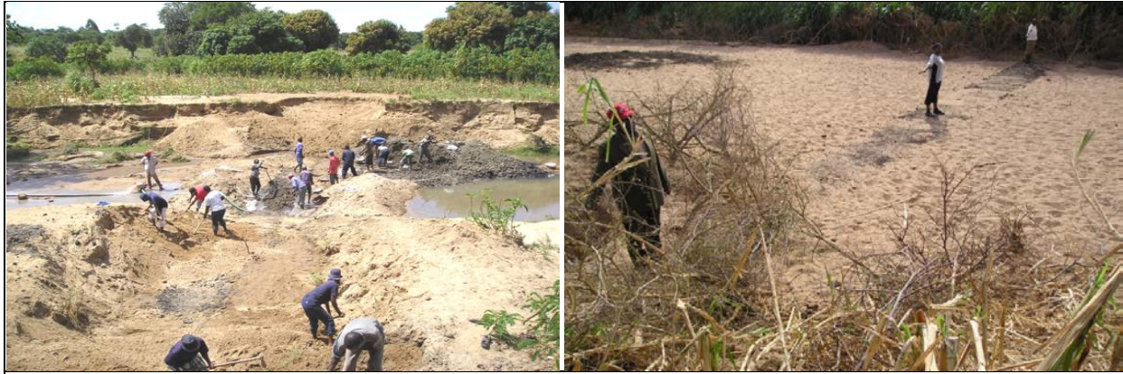
Subsurface dams: Left: under construction, Right: after the construction
