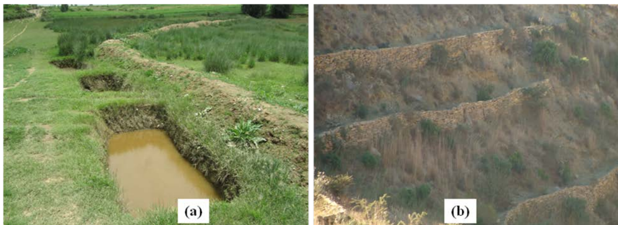
Plate 4: (a) Soil faced trench bunds, and (b) Stone faced trench bunds.
