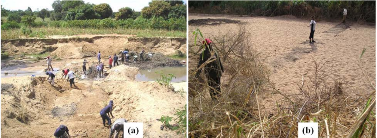
Plate 9. Subsurface dams: (a) under construction, (b) after the construction.
