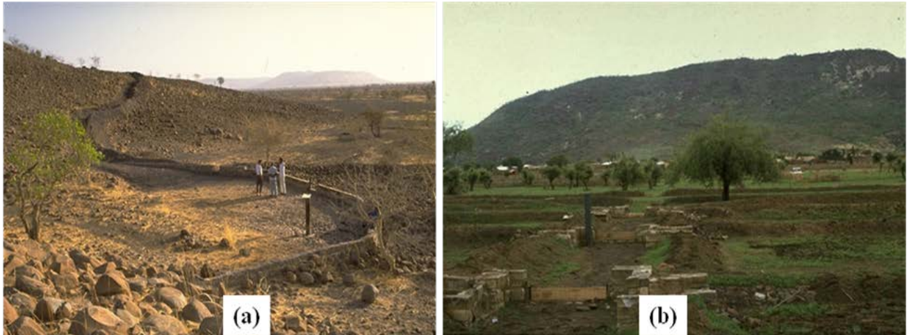
Plate 5: (a) Catchment area of hillside conduits, and (b) Conveyance Channel.
