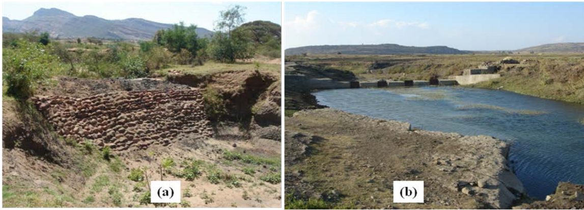
Plate 7. Check-dams: (a) Earthen Check-dam, (b) Concrete/Masonry Check-dams.
