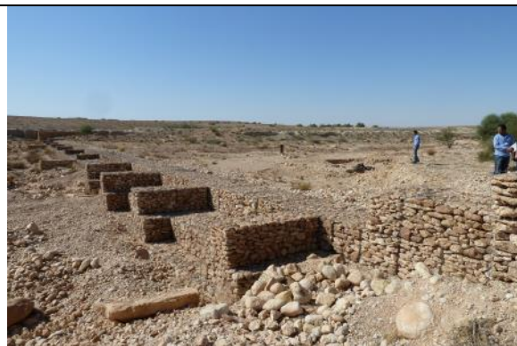
Fig 1. Gabion check dam with recharge well
