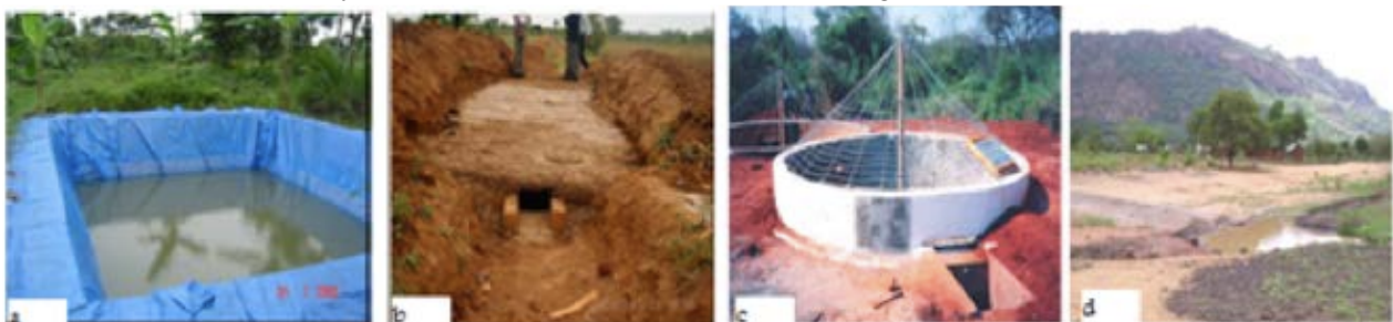
a. Underground rectangular plastic lined tank; b. A dead level contour with a Manama infield tank; c. An underground tank being built; d. A water pan on a natural depression
