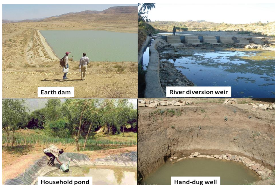
Figure 8 Some of the water harvesting technologies used for irrigation in the study area
