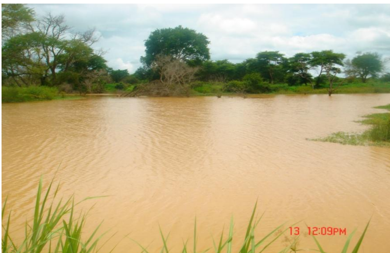
Dam at confluence of Magoye river and Ngwezi stream (13.01.2012)
